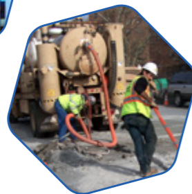
MicroTrench Installations
